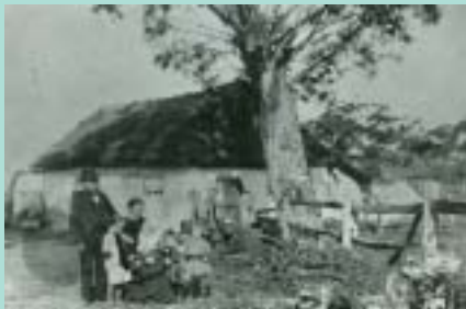
This photo shows a typical early German cottage in the Barossa. The walls are made of 'pug' (a mixture of clay and straw), and the roof is thatched straw. Note the post and rail fence on the right, using the gum tree as a post! Building verandas onto these cottages only became apparent after living through some hot Australian summers. Unfortunately the house, built c1860, and the family are unidentified. Barossa Valley Archives & Historical Trust
