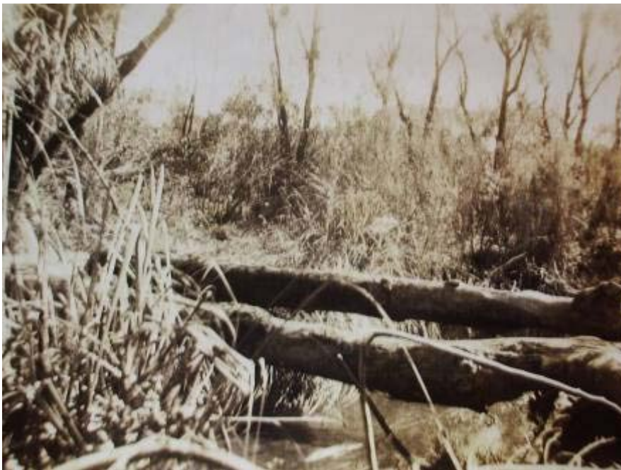
The start of a settler's 'corduroy' road over a stream, south-west Kangaroo Island (Courtesy of Joy Wheaton).
