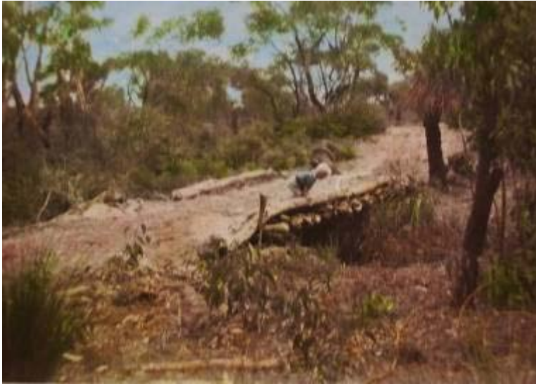
Completed road. About 1947 (Courtesy of Joy Wheaton)
